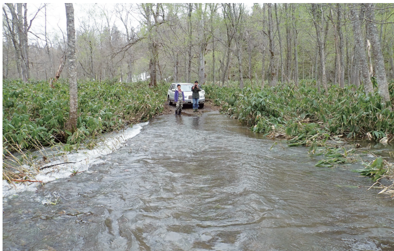
▲雪解け氾濫で林道が水没
